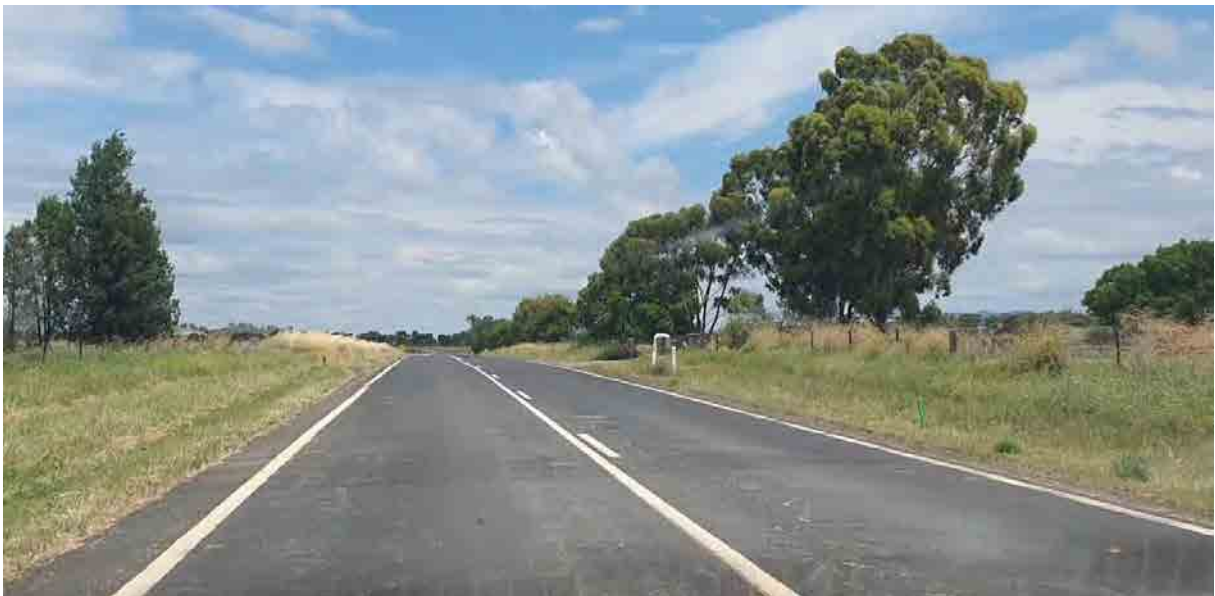
Figure 2.9: Goolma Road Street View (looking south)
