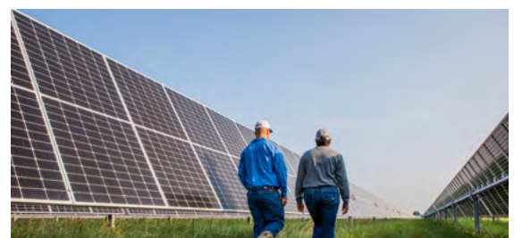
As they follow the sun during the day, solar panels reach a max height similar to a field of corn
