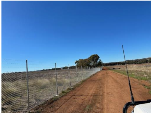
Photo 17: Perimeter fence and access road.
