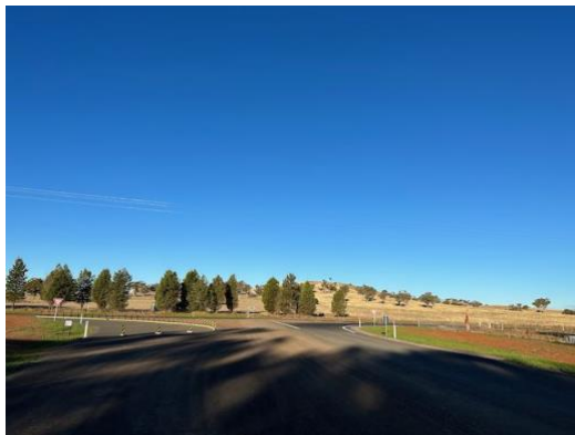
Photo 21: New access road and road upgrade.
