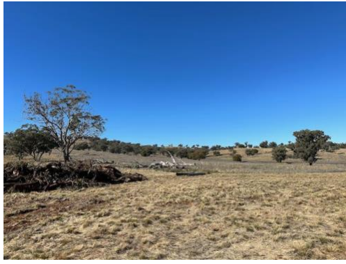
Photo 25: Clearing and grubbing along Transmission line.
