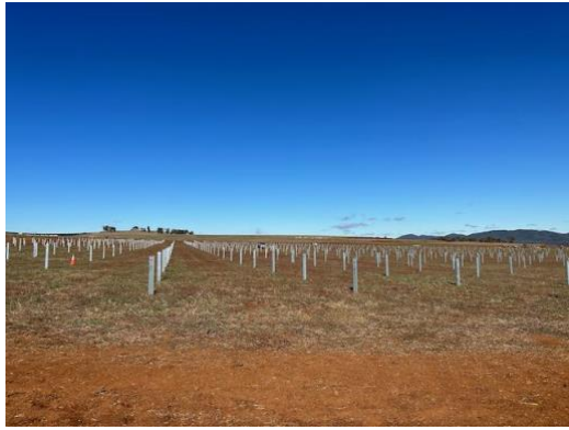
Photo 9: Indication of current stage of works – piling in some areas.
