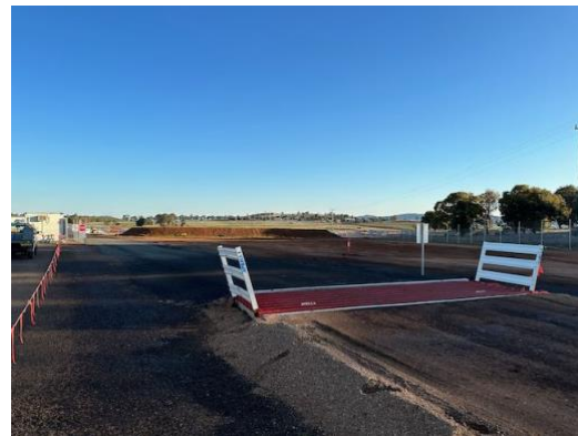
Photo 22: Rumble pad at main site access point.
