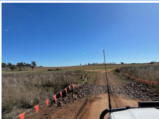
Photo 15: Evidence of temporary creek crossing at a designated point.
