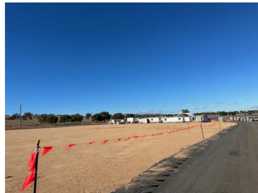
Photo 6: Laydown areas & all-weather access road.
