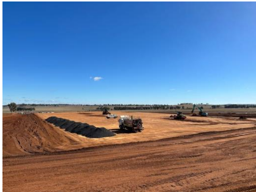
Photo 11: Works in progress at substation pad.
