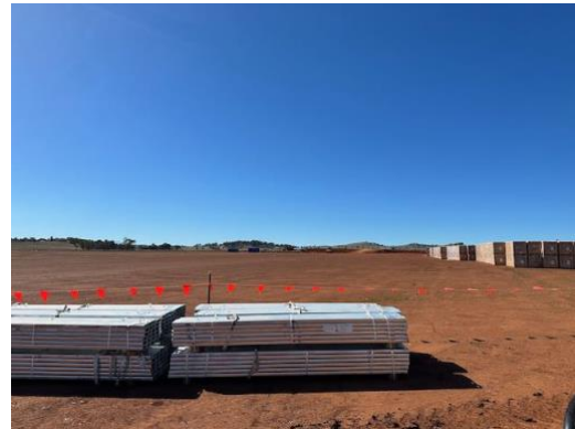
Photo 12: Evidence of materials in designated laydown location.
