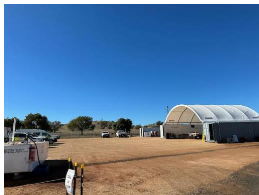
Photo 7: Site compound and maintenance areas.
