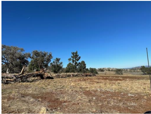
Photo 27: Clearing and grubbing along Transmission line. Course woody debris maintained.
