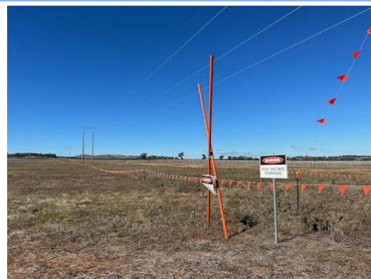
Photo 14: Evidence of exclusion zone below overhead transmission line.
