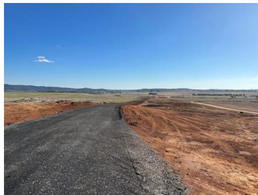
Photo 32: Evidence of all-weather access road to substation pad.
