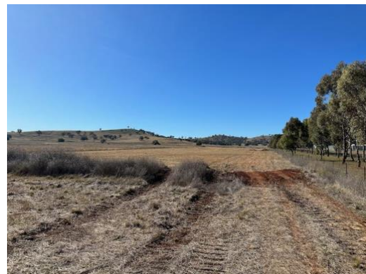
Photo 26: Transmission line route, view away from Goolma Road.
