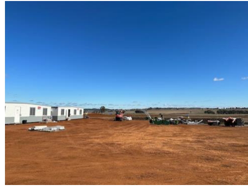
Photo 10: Substation pad site establishment.
