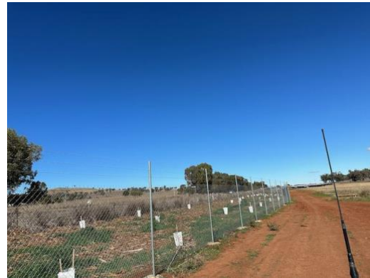
Photo 20: Perimeter fence and landscape plantings.
