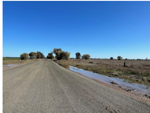
Photo 28: General condition of Blands Lane.
