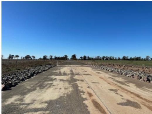
Photo 27: Causeway on Blands Lane. Road upgrade not yet completed.
