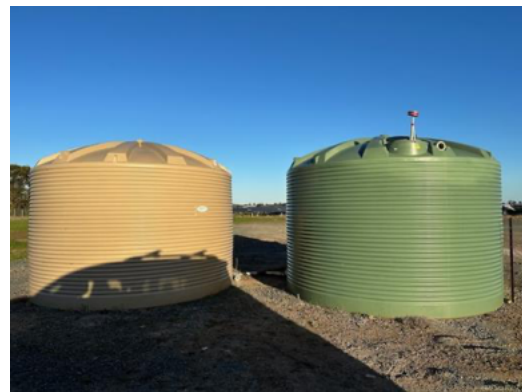
Photo 14: 2 x 22,500L water tanks for fire-fighting purposes.
