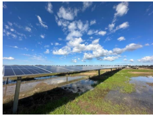
Photo 18: General site conditions.
