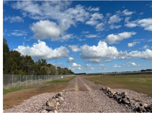
Photo 2: Main site access track with low spot stabilised crossing.
