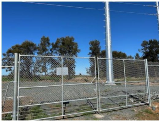
Photo 25: Myers Lane access gate.
