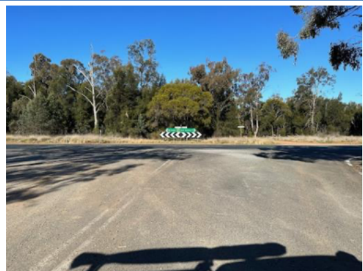
Photo 32: Bodells Lane and Newell Highway intersection.
