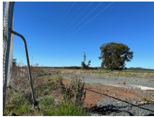
Photo 26: Clearing completed in Myers Lane
