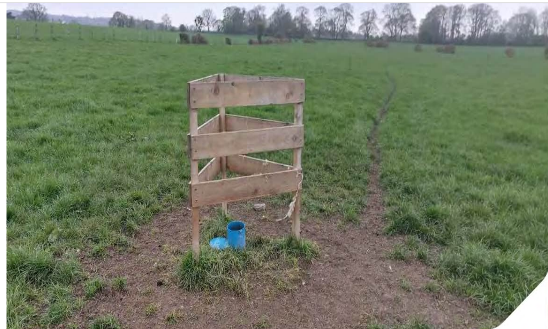
Plate 08: Southern parcel – Borehole monitoring standpipe in the north-east
