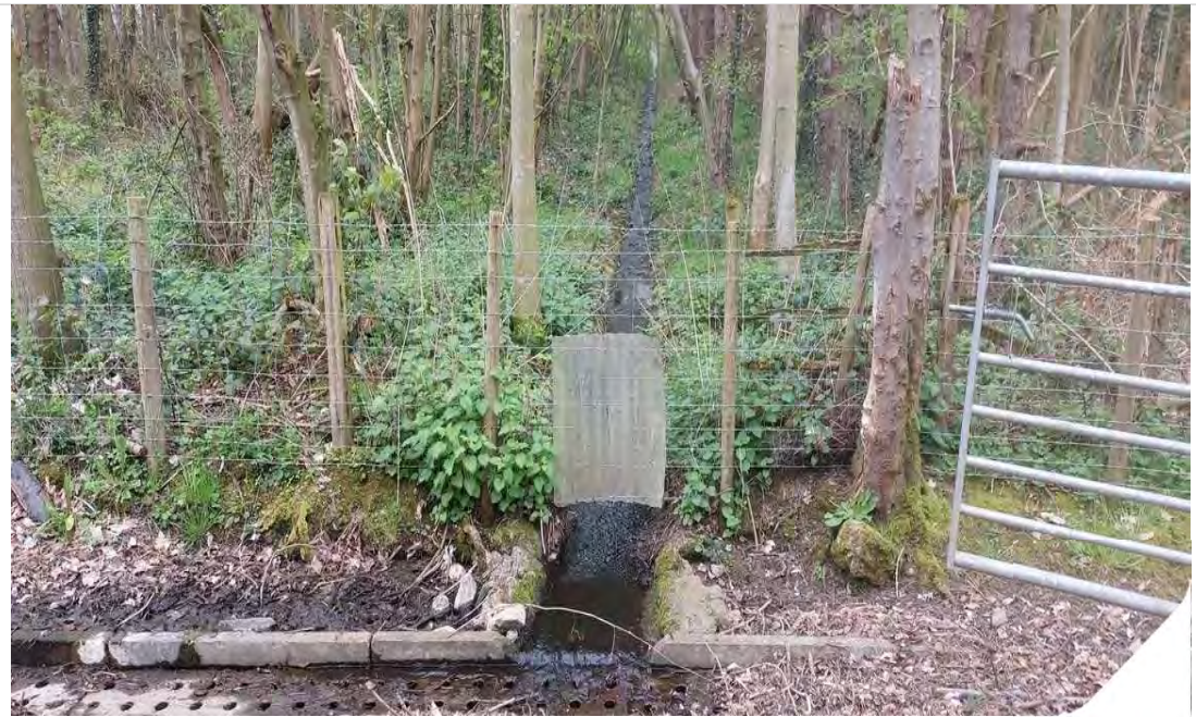
Plate 02: Southern parcel – Drainage channel from off site pond
