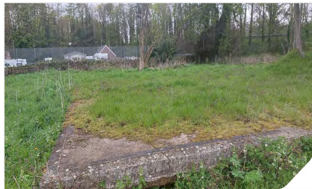
Plate 09: Southern parcel – Foundations of former building in the east of site
