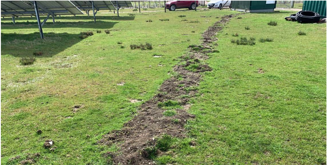
Insert 47: Trench During Wet Period (example from Bedfordshire)
