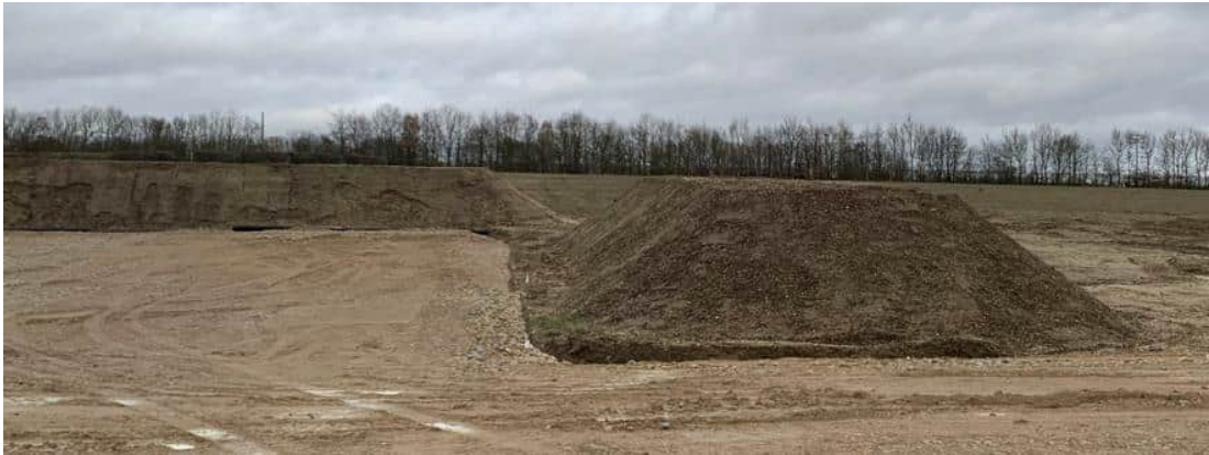
Insert 14: Topsoil Storage Bund (example from Lincolnshire)
