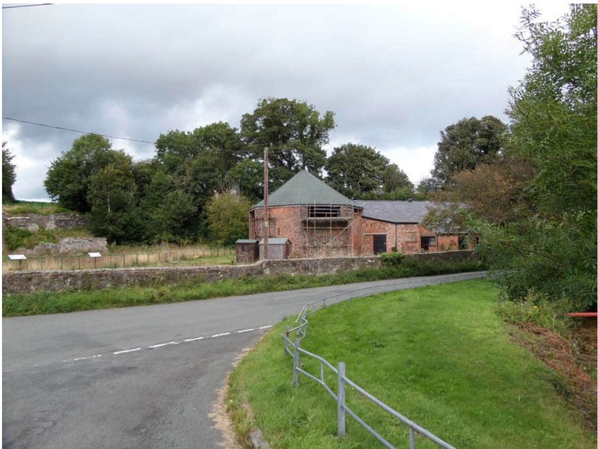
Plate 32: Bersham Ironworks remains from the south
