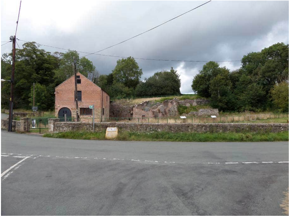
Plate 33: Bersham Ironworks remains from the south
