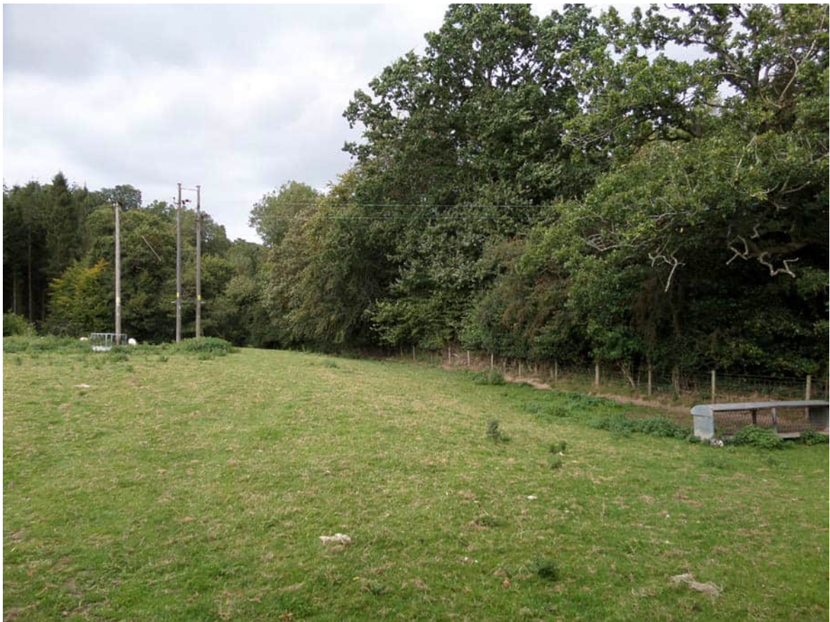
Plate 44: View north along the section of Offa's Dyke running through Plas Power woods, to the west of zone D – the line of the Dyke is marked by the dense trees on the right of the picture
