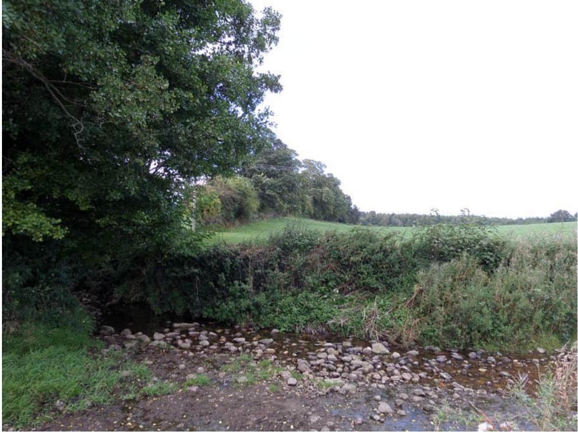
Plate 43: View north along section of Offa's Dyke to west of zone F
