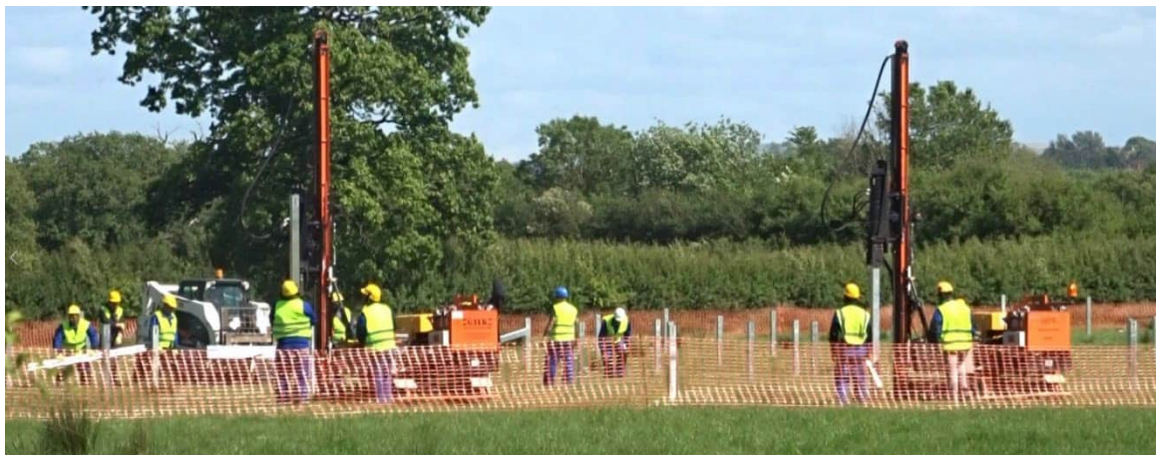
Photo 10.2: Example of Solar PV Leg Installation
