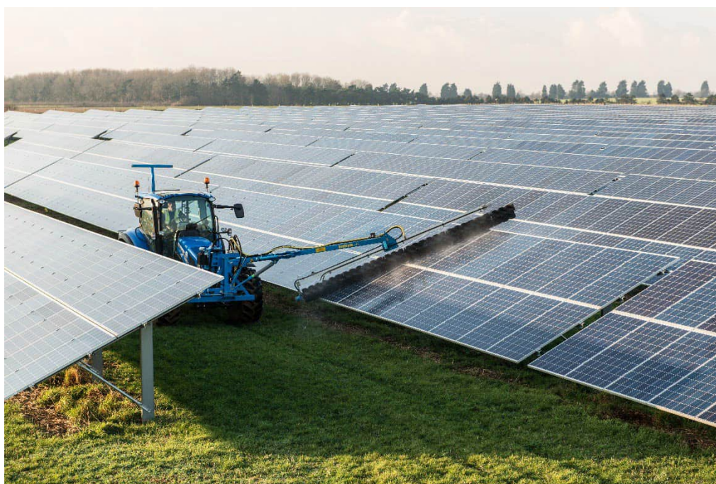
Image 6: Example of solar array maintenance at existing operational solar site
