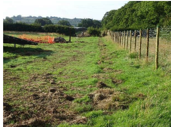
Insert 52: Topsoil Replaced
