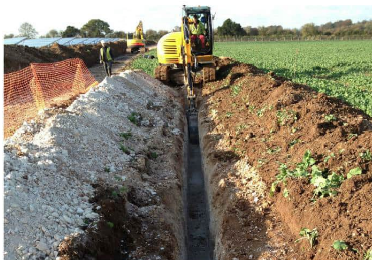
Insert 53: Machinery Used for Trenching
