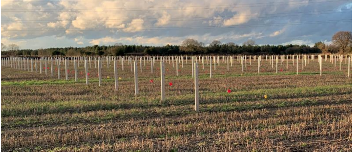
Image 12-3 Piles for Solar PV Tables
