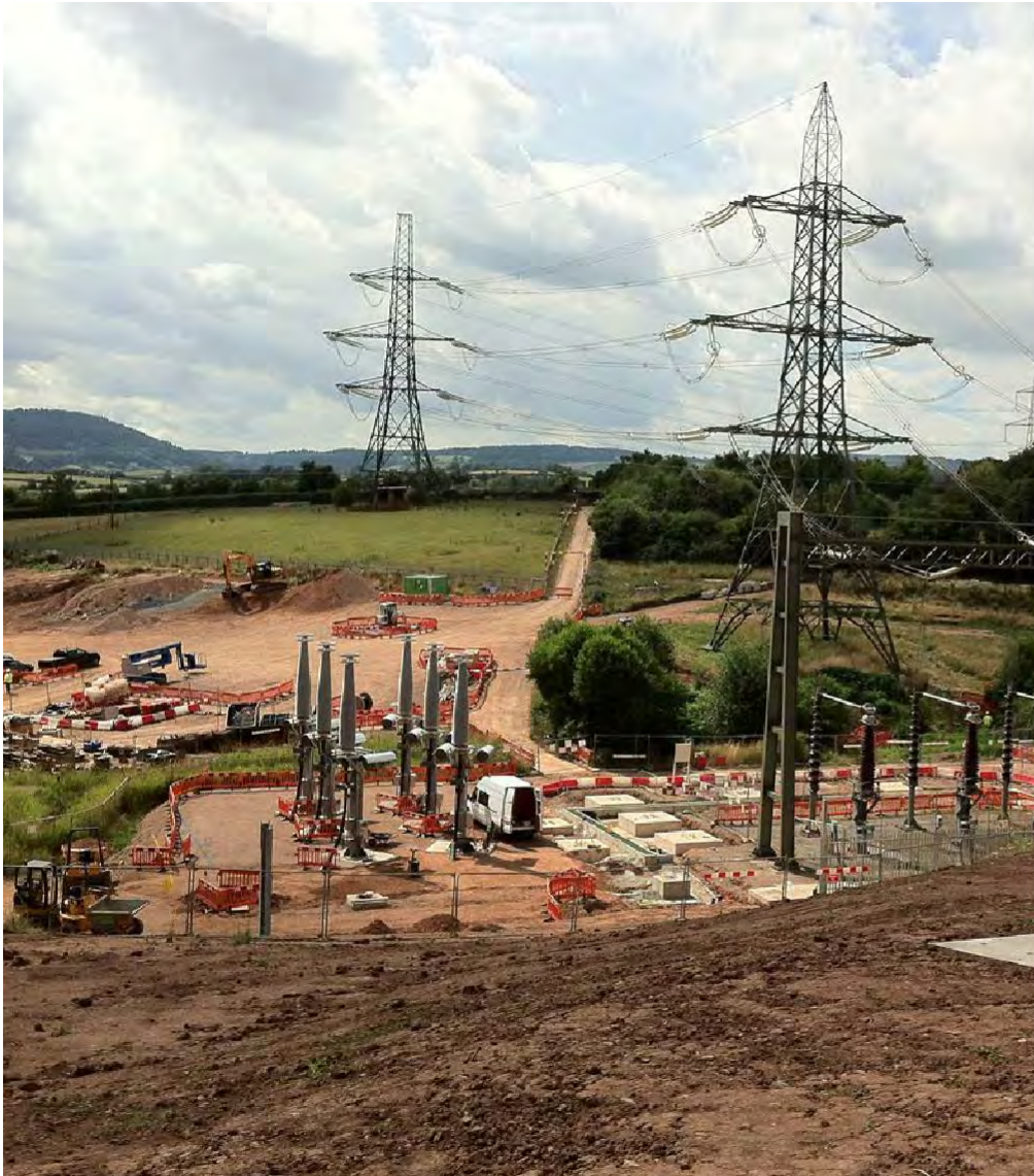
The undergrounding of electricity cables at Ross-on-Wye
