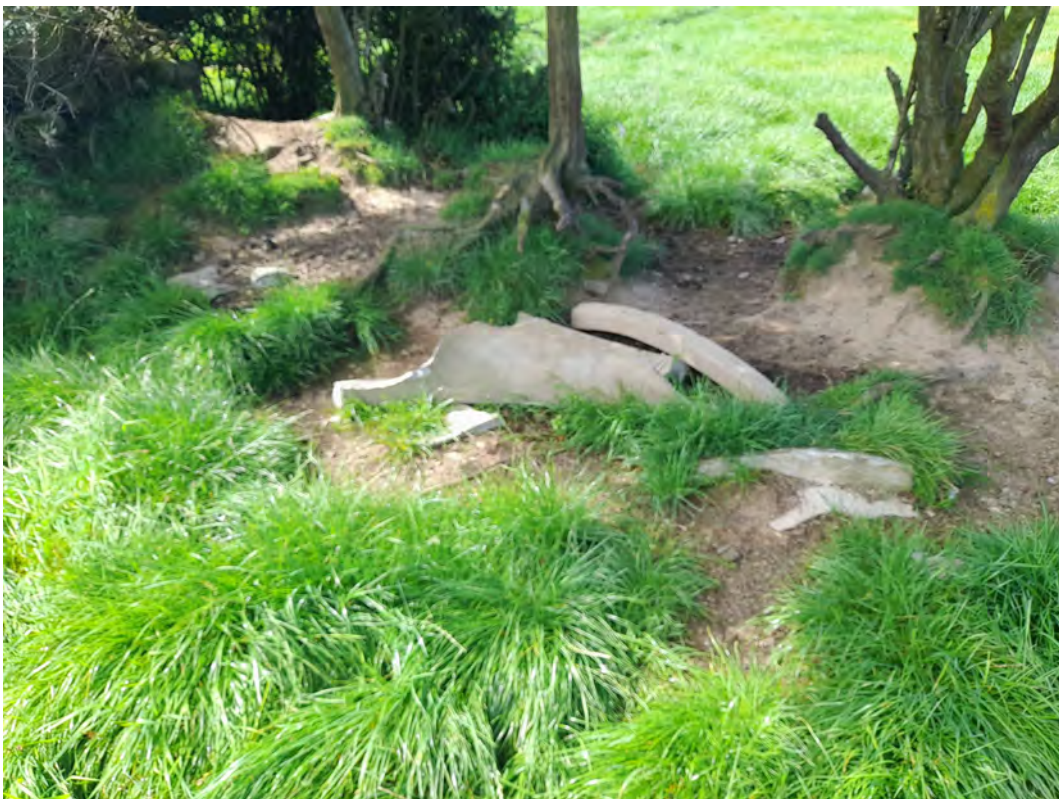
Photo 4—Possible asbestos identified along boundary near to farm buildings within north east of area.
