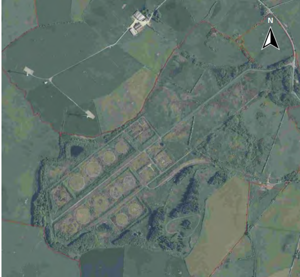
Figure 2:2: Aerial Photograph of Former Oil Storage Depot
