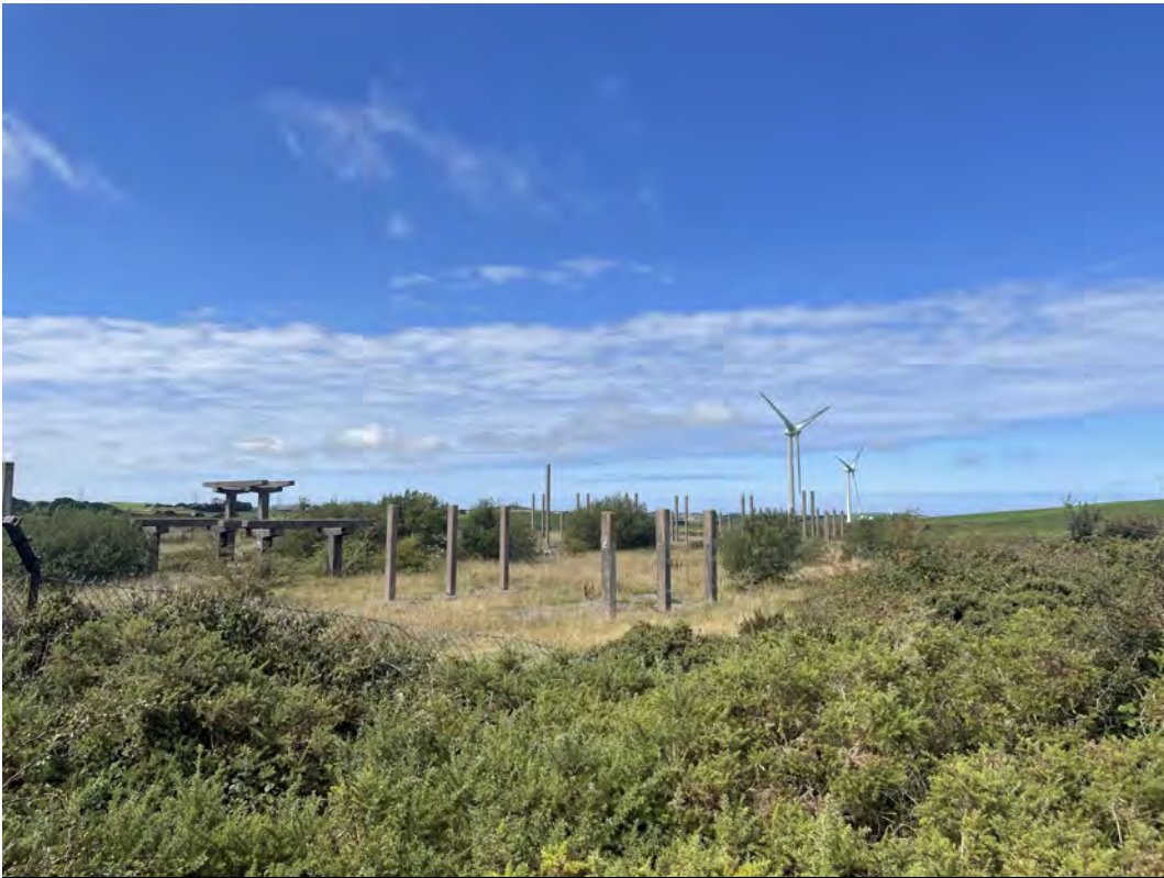
Photo 7—Remnant infrastructure within former oil storage terminal.
