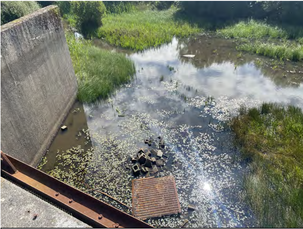
Photo 11—Drainage infrastructure within south west of site.
